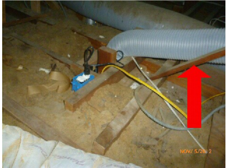
Damaged duct in attic
