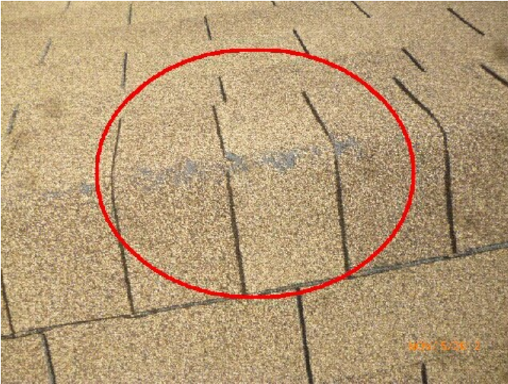
Roof surface deteriorating
