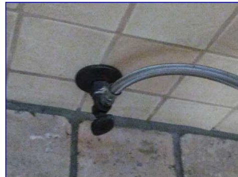
Corroded plumbing
