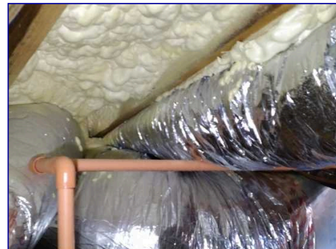
Restricted, crushed
