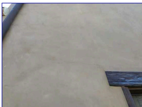
Cracks rear
