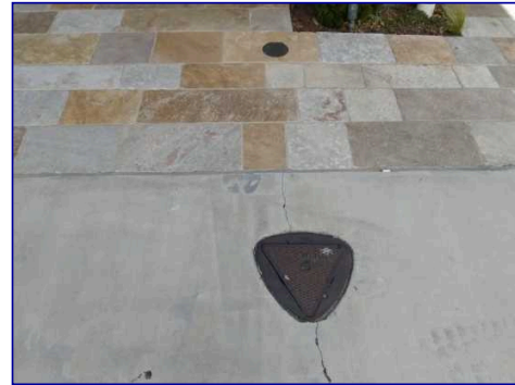
Clean out driveway
