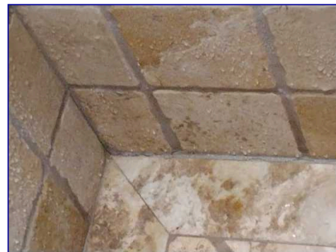
Poor grout
