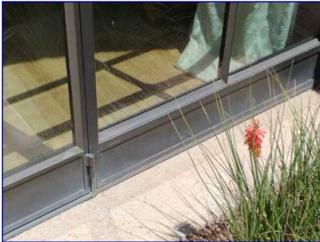
Front right weathered
