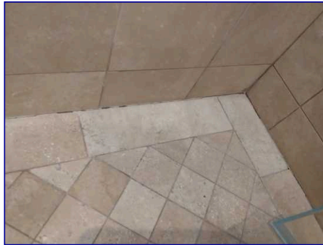
Poor grout
