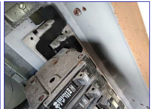
Bus corroded
