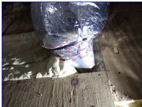
Missing insulation
