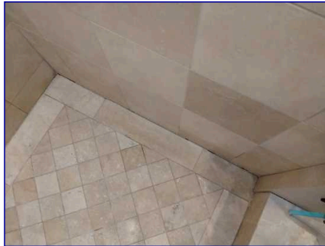
Poor grout
