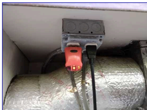
Exterior no gfcf
