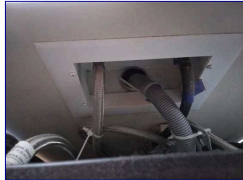
Corroded plumbing
