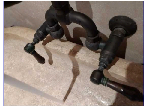
Corroded fixture
