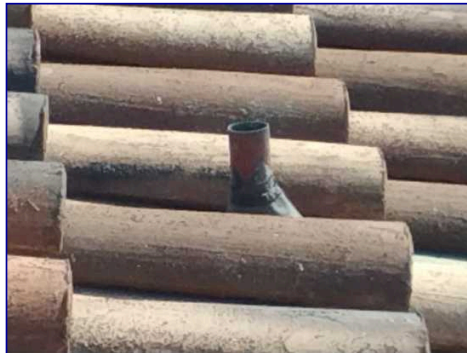
Mastic cracking
