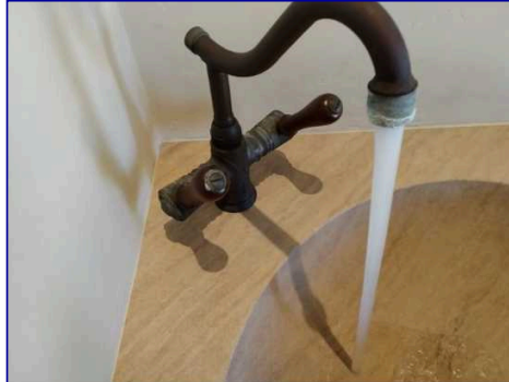
Corroded fixture
