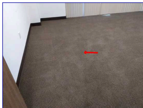
Sloping front office
