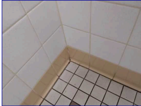
Grout cracks
