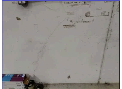
Cracks, efflorescence
