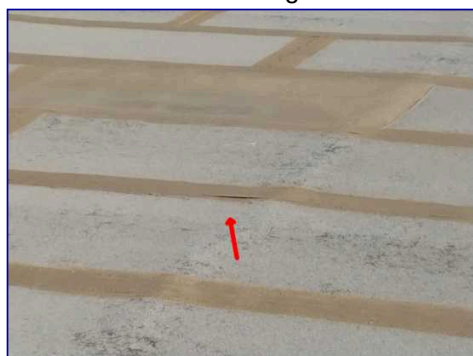
Joint cracks
