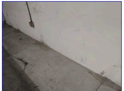
Cracks, efflorescence
