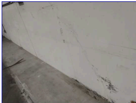
Cracks, efflorescence
