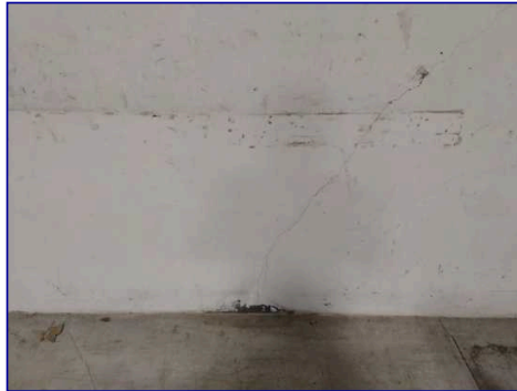
Left cracks,efflorescence
