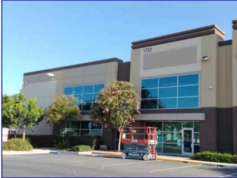
The front of the building
