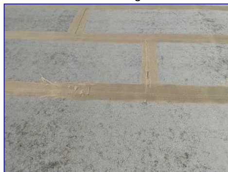
Joints cracks
