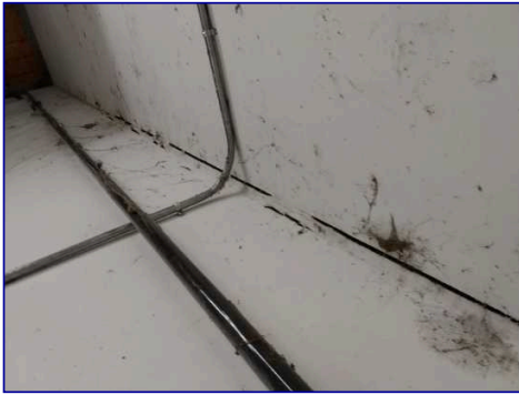
Joints cracks
