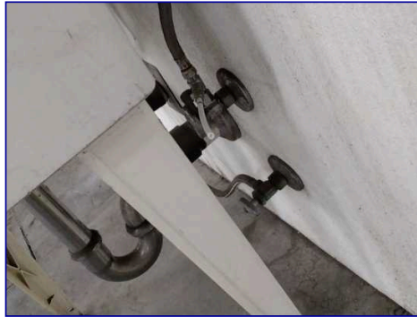
Warehouse sink plumbing corroded
