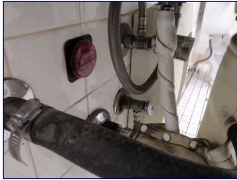
Corroded plumbing
